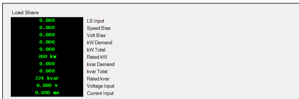
Figure 4-148. Metering Explorer, Diagnostics, Load Share Screen
