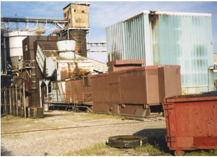
Figure 1: Combustion Turbine Generator
