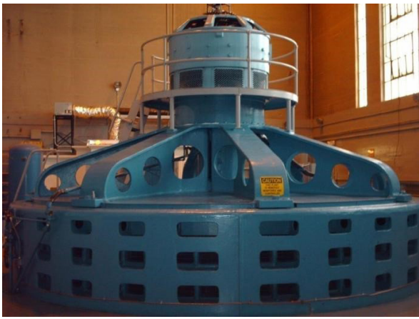
Figure 2. Salient-Pole, Vertical-Shaft Hydro Machine
