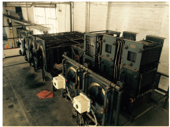
Figure 5. Wire-Wound Rheostat (one per machine)
