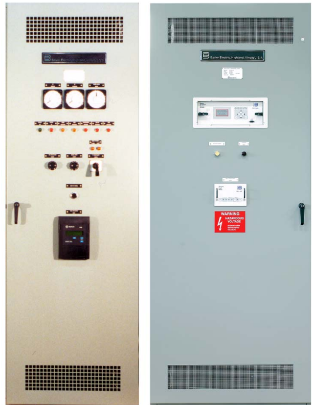
Fig. 1. A Comparison of an Analog-Controlled Excitation System (left) and an Integrated, Digitally Controlled Excitation System (right)
